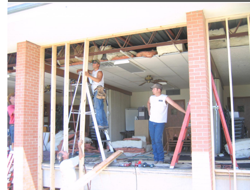
Work on remodel of South rooms begins.
